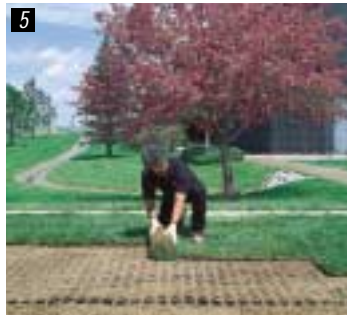
5 Hydroseed or lay sod.
