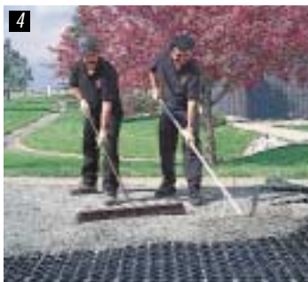
Fill rings with clean gravel.
